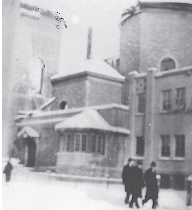
St. Joseph's Rectory after the fire. Rectory suffered only water and smoke damage. December 28-31, 1930.
