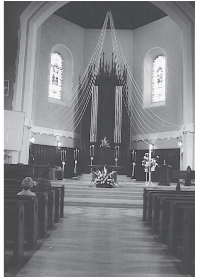
Interior of third St. Joseph's Church after the first series of structural changes made to its structure. Circa 1982.
