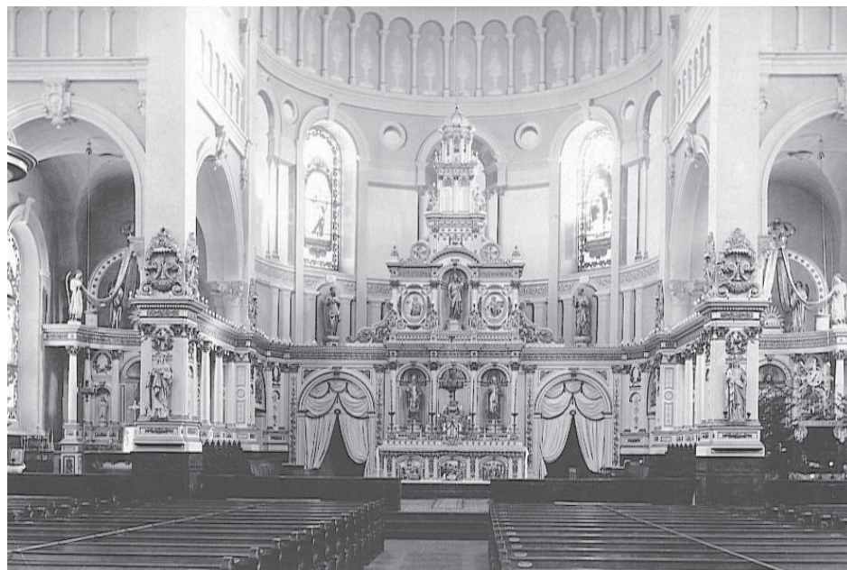
Interior view of second St. Joseph's Church 1915 -1930. Photo credit, Archives Deschâtelets – Photographer unknown
