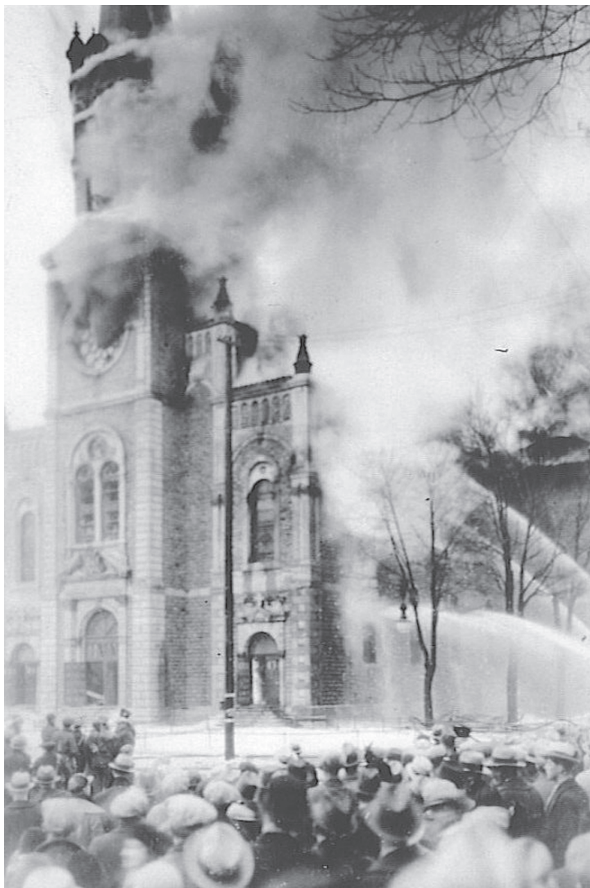
St. Joseph's Church burning. About twenty minutes after this photo was taken, the steeple fell inward onto the roof, collapsing what remained of it. December 27, 1930.
