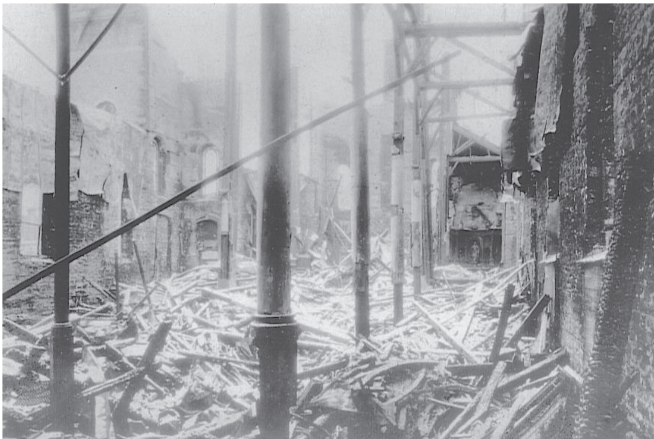
St. Joseph's Church after the fire. Note the statue of the Sacred Heart of Jesus still standing in the middle right side of this photo. December 28-31, 1930. Photo credit , Archives Deschâtelets – Photographer unknown.
